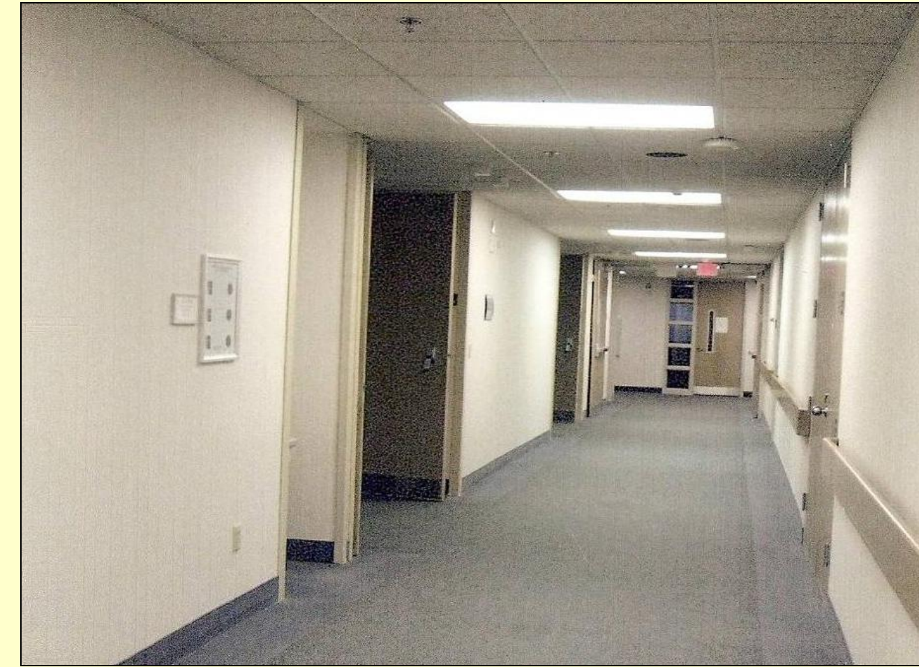
Unit hallway prior to renovation
